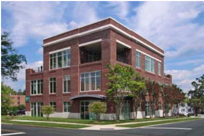
Bragg Building 1031 South Caldwell Street, Charlotte
