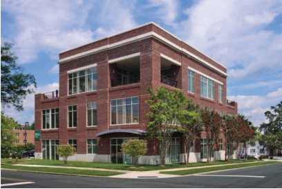
Bragg Building 1031 South Caldwell Street, Charlotte
