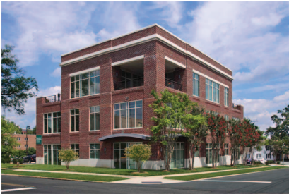
Bragg Building 1031 South Caldwell Street, Charlotte
