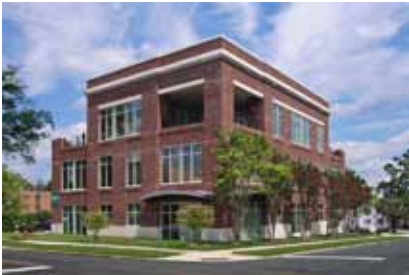
Bragg Building 1031 South Caldwell Street, Charlotte
