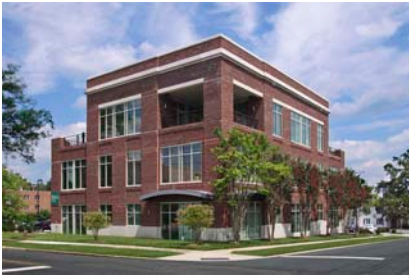
Bragg Building 1031 South Caldwell Street, Charlotte
